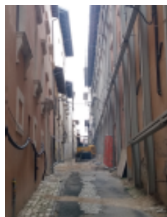
Figure 2. Reconstruction continues in L'Aquila, Italy. A side street off the main thoroughfare. Buttressing on the buildings on the right-hand side of the alley. Credit: Julie Dugdale, October 2019.
