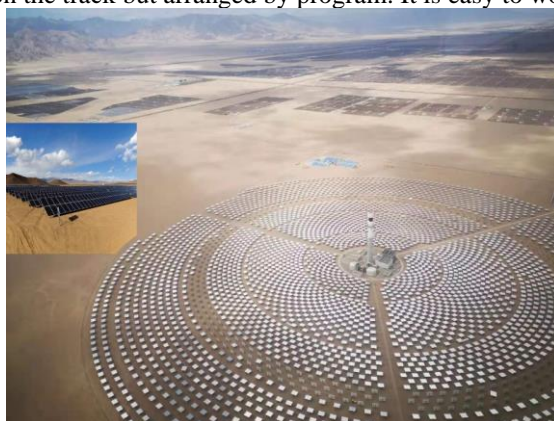
Source: Taken from North-West of China. Figure 1: Solar power station.
