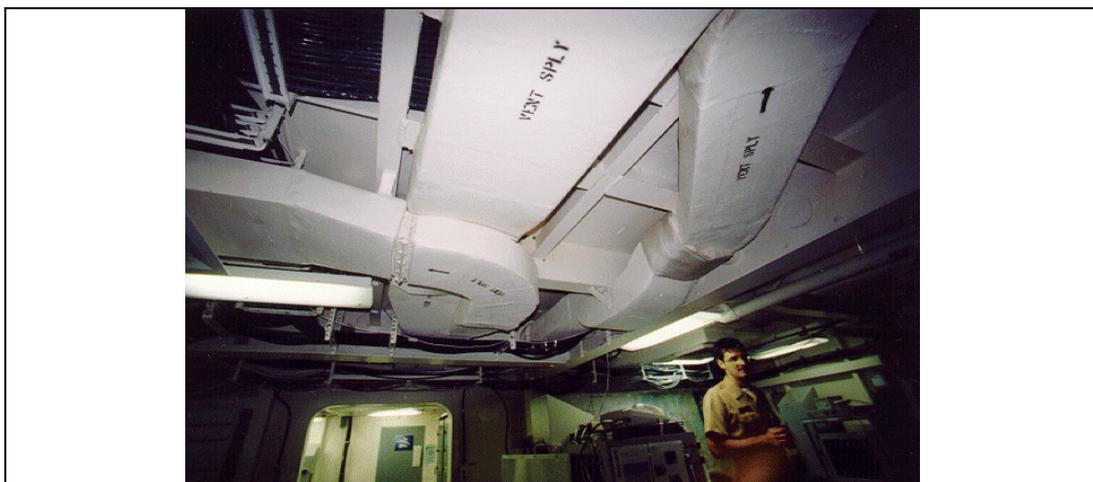
**Figure 1** An example of snaking ventilation shafts in the Joint Air Operations Center aboard the USS CORONADO
